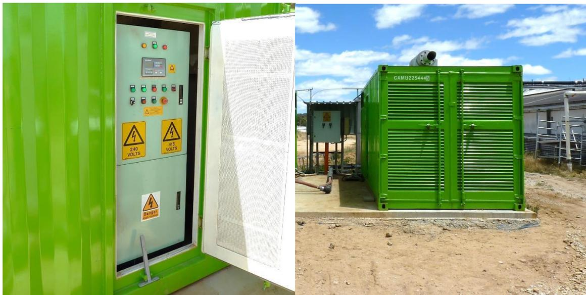
Figure 2.4 Emergency switches located outside an on-farm generator skid
