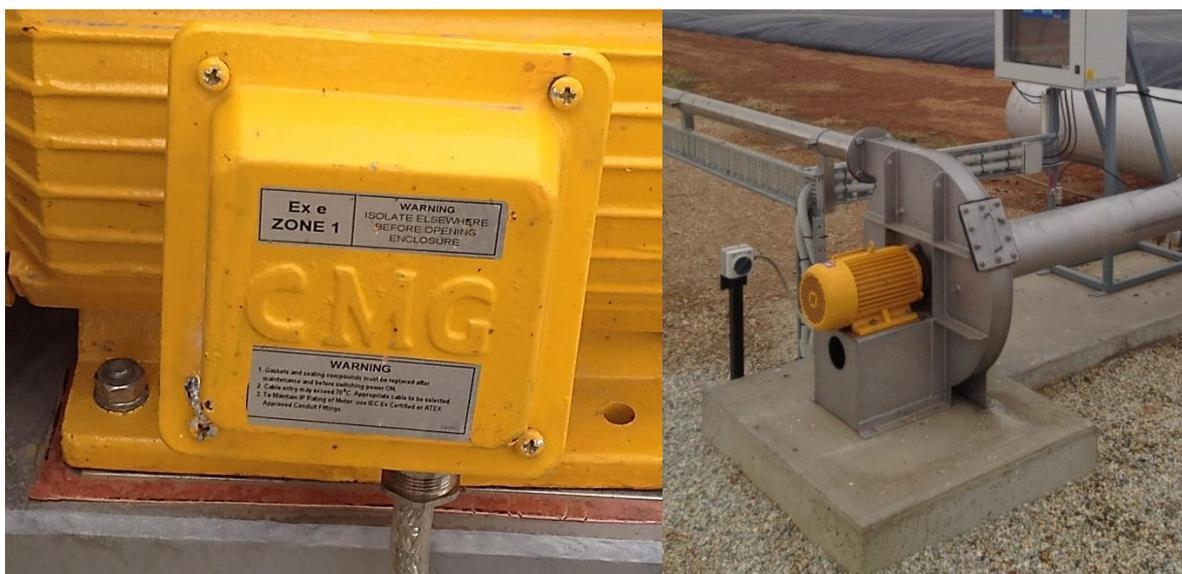
Figure 2.2 Example of a biogas blower at an Australian piggery rated to Zone 1
