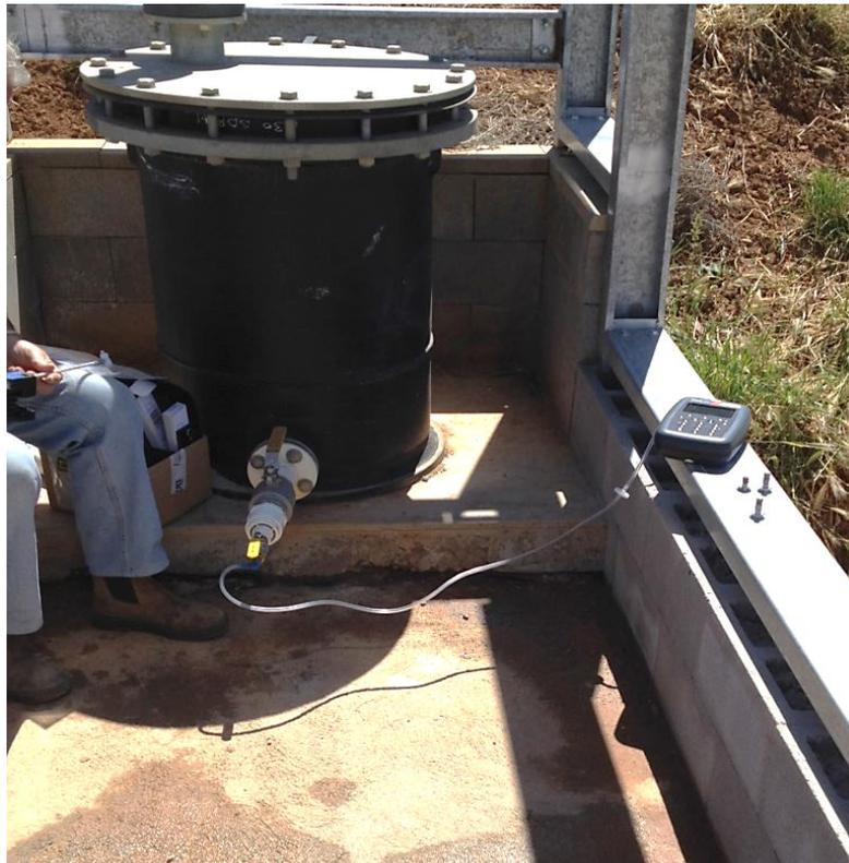
*Figure 3.1 Measurement of biogas composition on-farm can confirm whether explosive gas mixtures have successfully been purged from biogas equipment and piping. The biogas meters shall be appropriately rated for use in potentially explosive gas atmospheres (courtesy of the Pork CRC)*
