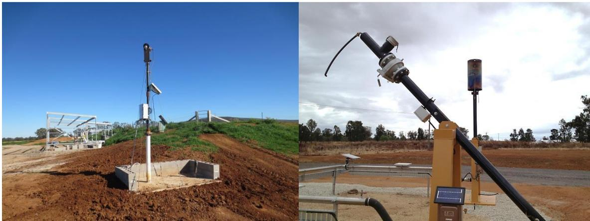
Figure 2.3 Typical on-farm biogas spark-ignition flares in Australia
